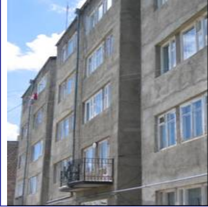
Ghandilyan Condominium The Gutter Pipes of the Project Building
