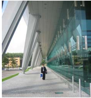
Janet Cohen walks along the outside of the ING Bank to get a better look at the stilt support system.
