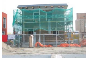
A strawbale house under construction in IJ Burg.
