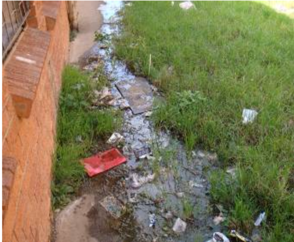
Blocked Sewer on School Property
